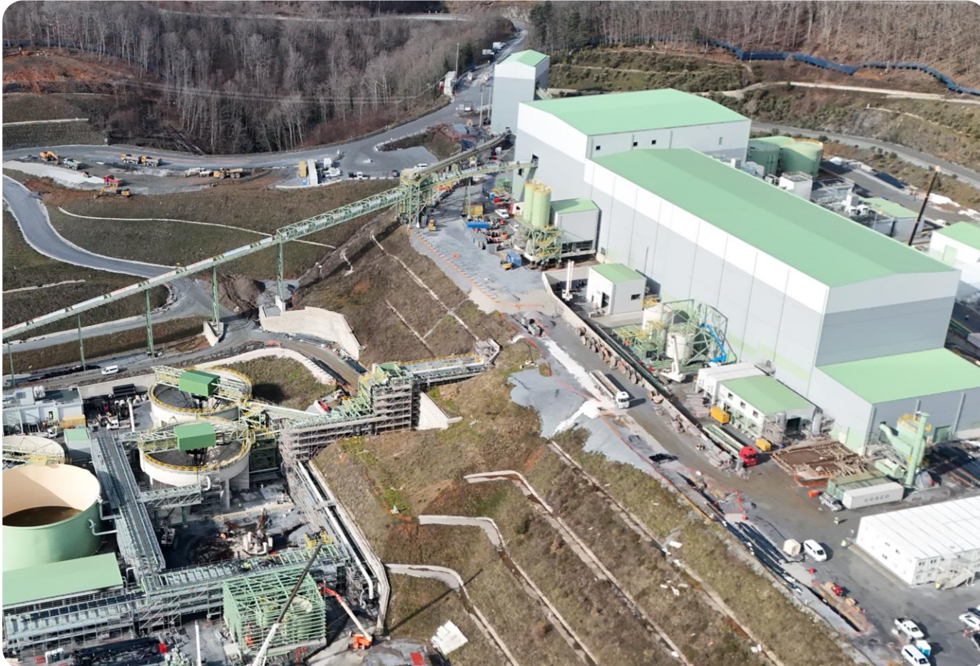
East side view of infrastructure
