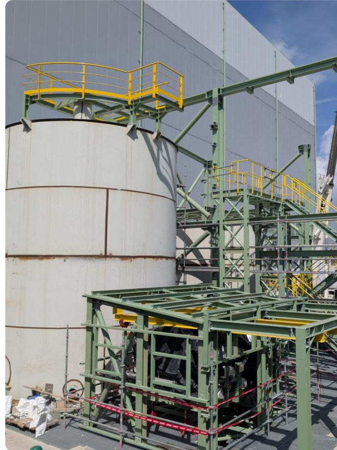
Guar building erection and pump skid
