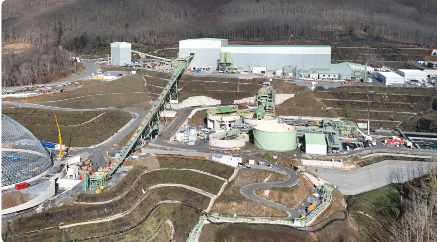
Aerial – process plant
