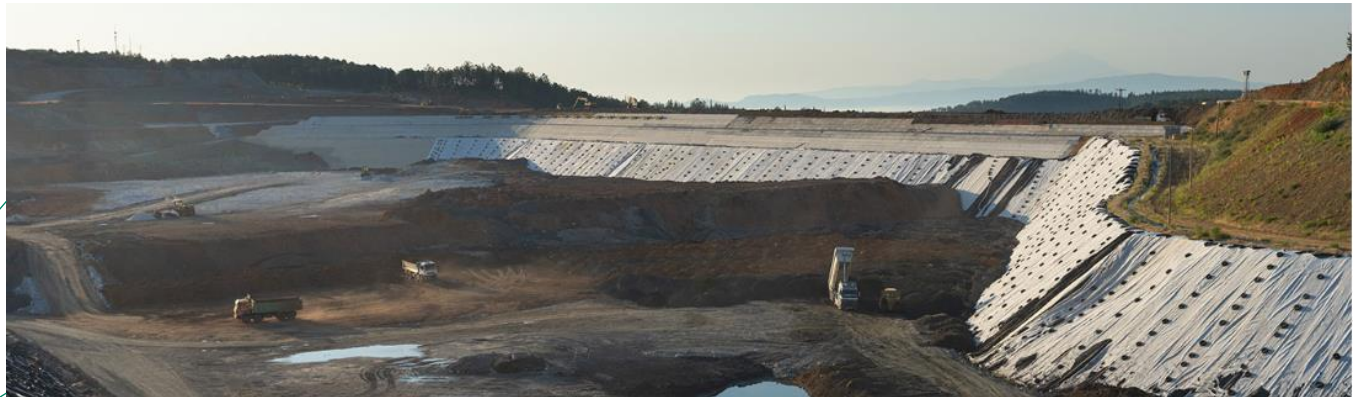
Kokkinolakkas filtered tailings facility
