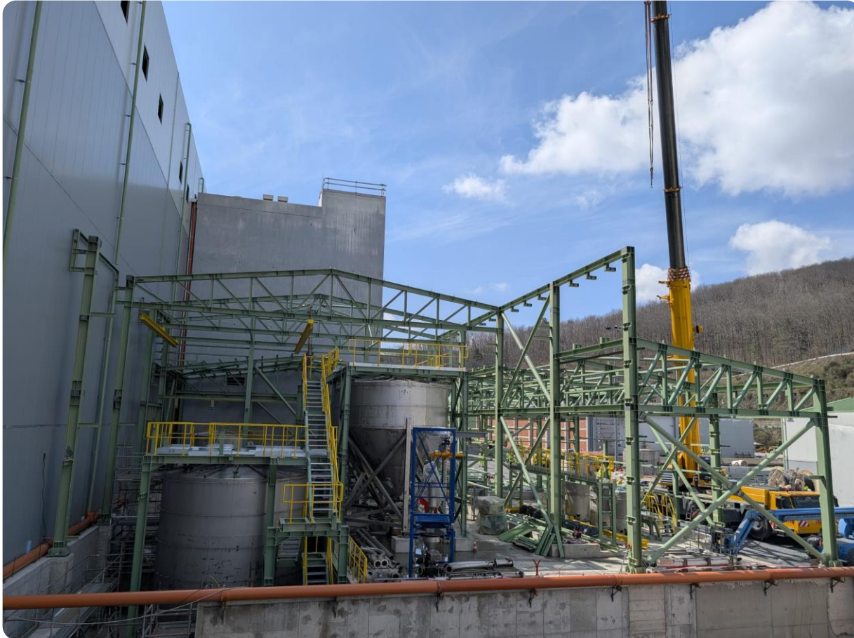
Sulphidizer building erection
