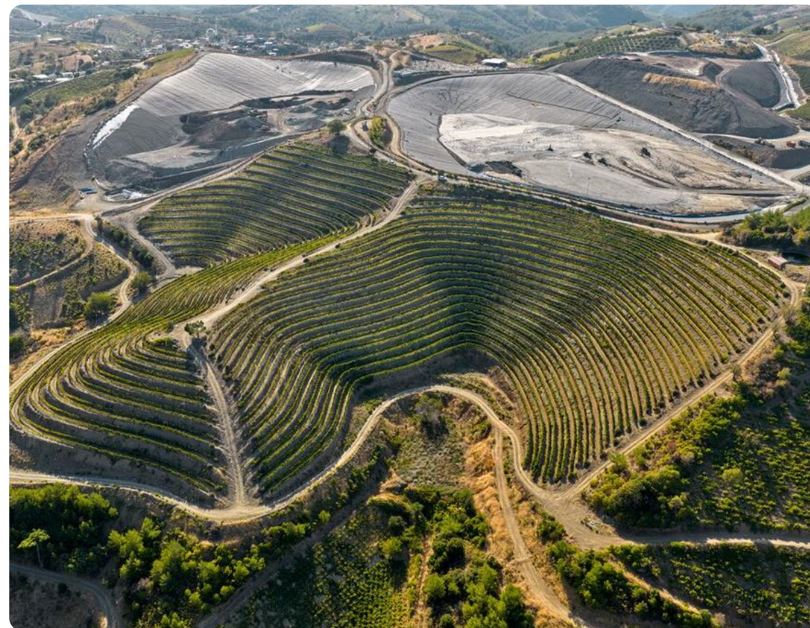
Efemçukuru – dry stack tailings and reclaimed area
