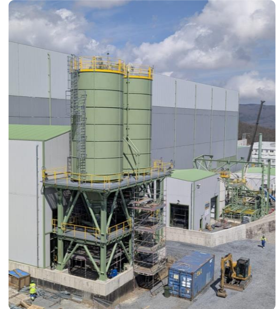
Lime, blower, compressor buildings
