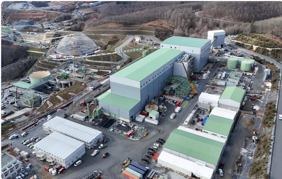
Process plant overview
